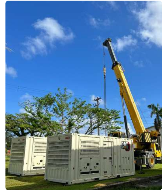
PFMD personnel assist in replacement of backup generators after Typhoon Mawar.
